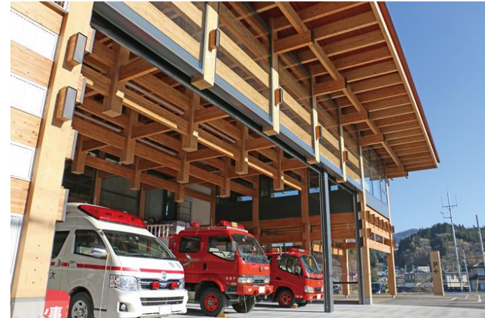
Sumita-town fire department building
